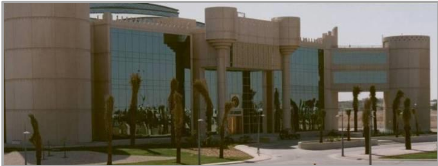
Air Defense Head Quarters Building
